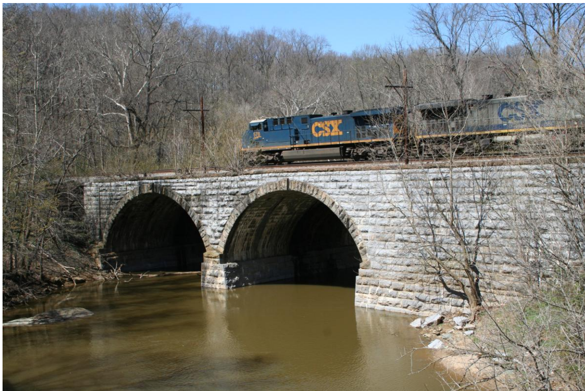
1902 side of B&O's Catocin Creek Viaduct. Photo by Richard Lind April 4, 2009
